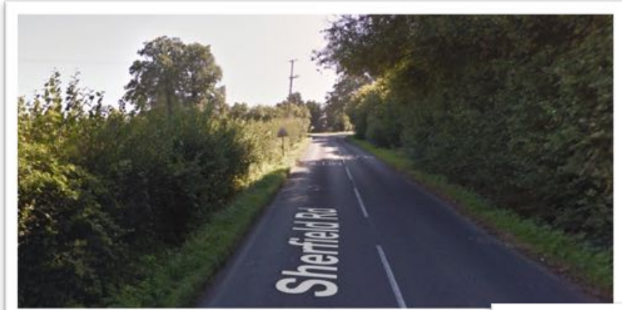
Figure 6 - Sherfield Road, C32 from Campbell Road towards Sherfield-on-Lodden
